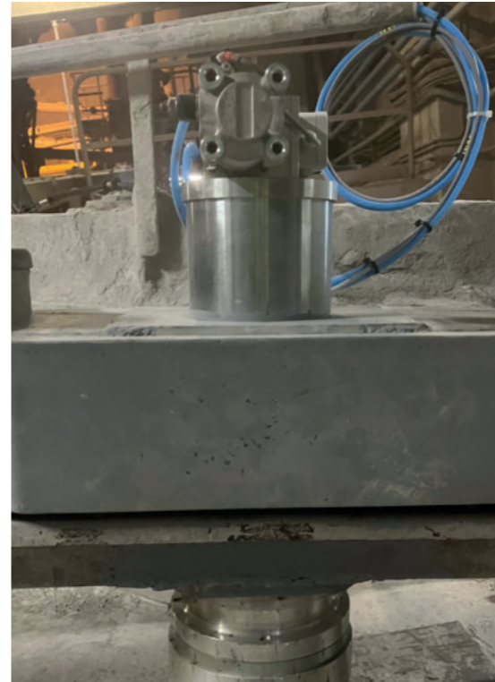
Installation on site
